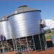
Above The use of inverted pullers and new drying bins installed by farmers helps to minimise aflatoxin
